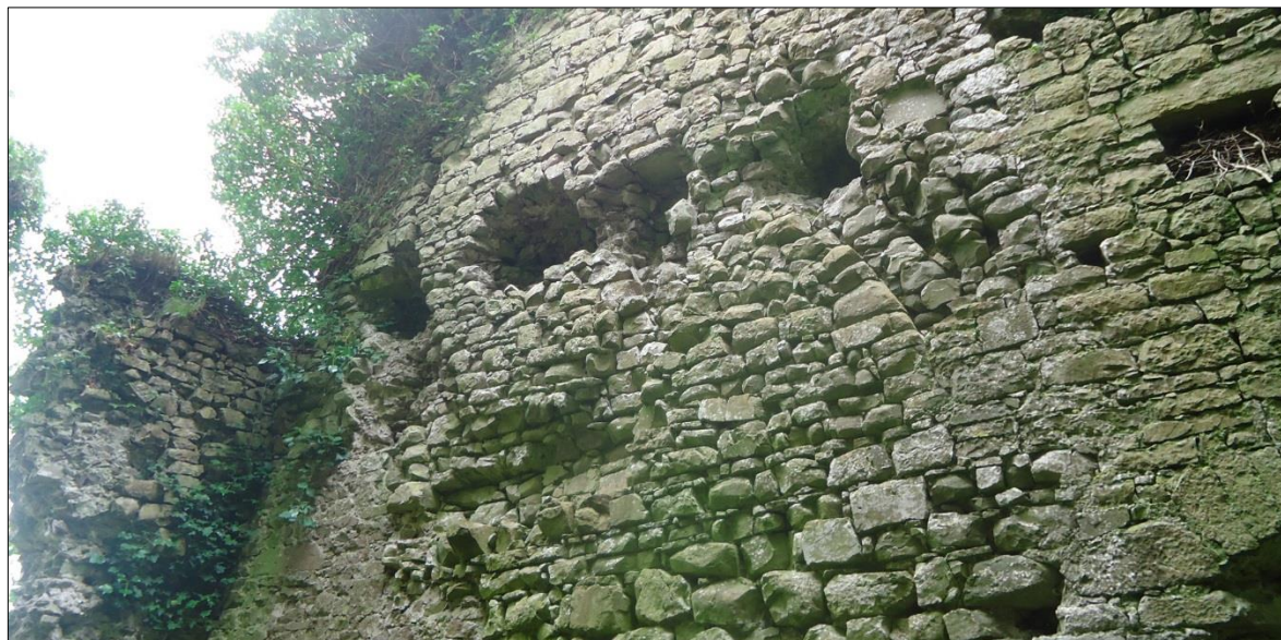
Plate 31: Ballintober Castle, southwest corner tower, view looking at the north side of the east wall, showing the arched recesses of the ground-floor ceiling, and a series of four recesses for joists above to support the a timber floor on the first floor. The absence of these elements on the right (south) side of the picture may indicate that this reflects rebuilding of the tower's interior at some point
