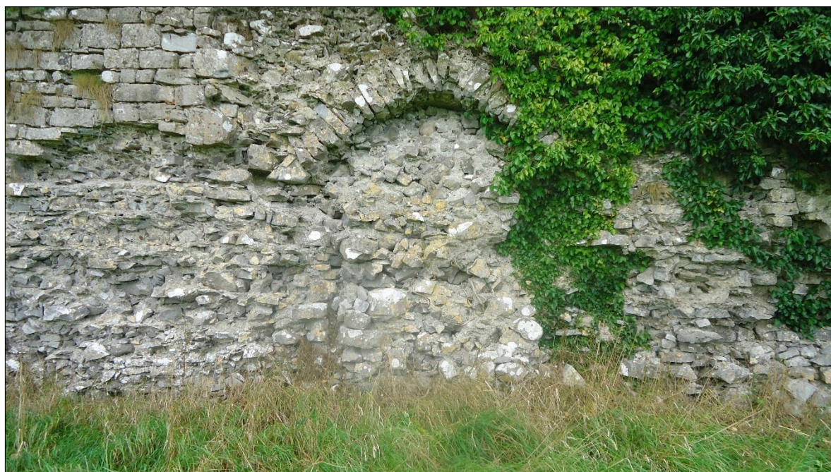
Plate 12: Ballintober Castle, view looking view at interior of west wall showing blocked-up window opening under arch
