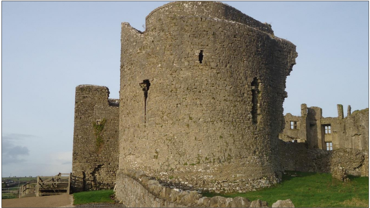
Plate 35: Defensive slit openings, Roscommon Castle. View shows the southwest corner tower with its tall narrow arrow slits, which (in common with those at Ballymote Castle, Plate 36) are noticeably taller and more defensible than those at Ballintober Castle
