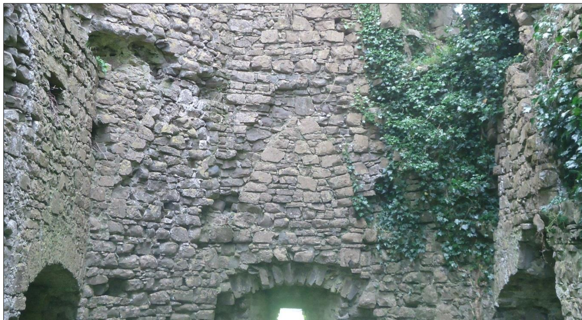
Plate 27: Ballintober Castle, southwest corner tower, view looking at the steeply-pitch arched recess above the south window, which served as one of several such arches to support a complex ceiling. Similar arched-recesses exist to the left and to right on the angled facades of the tower
