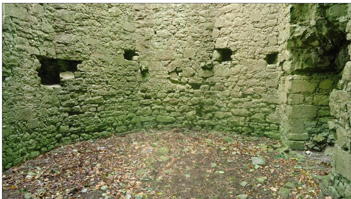
Plate 44: Ballintober Castle, northwest corner tower, view of the north end of the ground floor level, showing no indication of the blocked-up window openings discernible externally. The two squared recesses either side of the end-angle are to support joists for the floor level above
