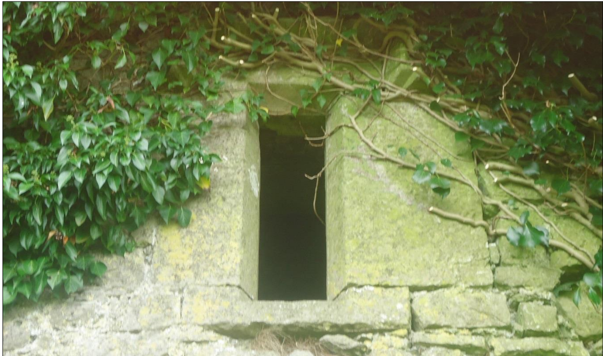
Plate 39: Ballintober Castle, northwest corner tower, view looking above entrance at mezzanine level to a short vertical opening with a flat hood moulding
