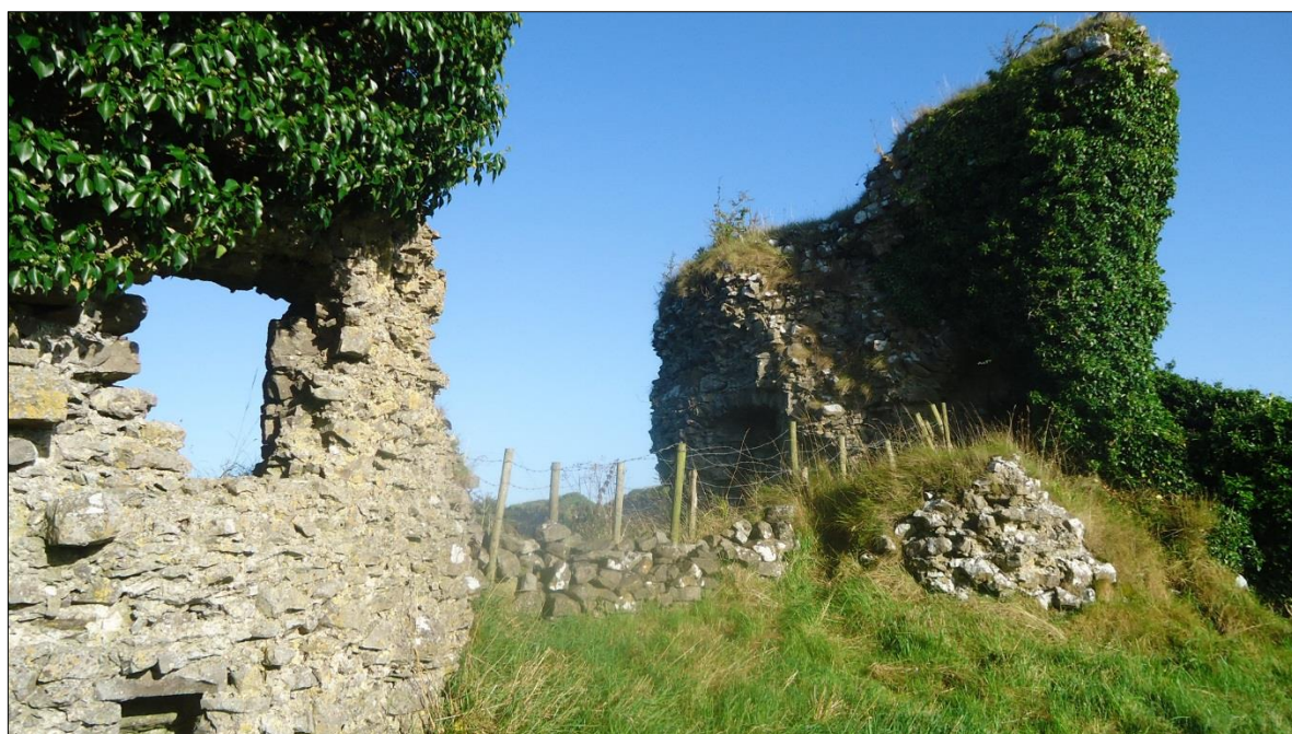
Plate 71: Ballintober Castle, eastern entrance, view looking north across entrance from the south tower to the north tower. The masonry mass in the foreground is the ruined base of the north tower
