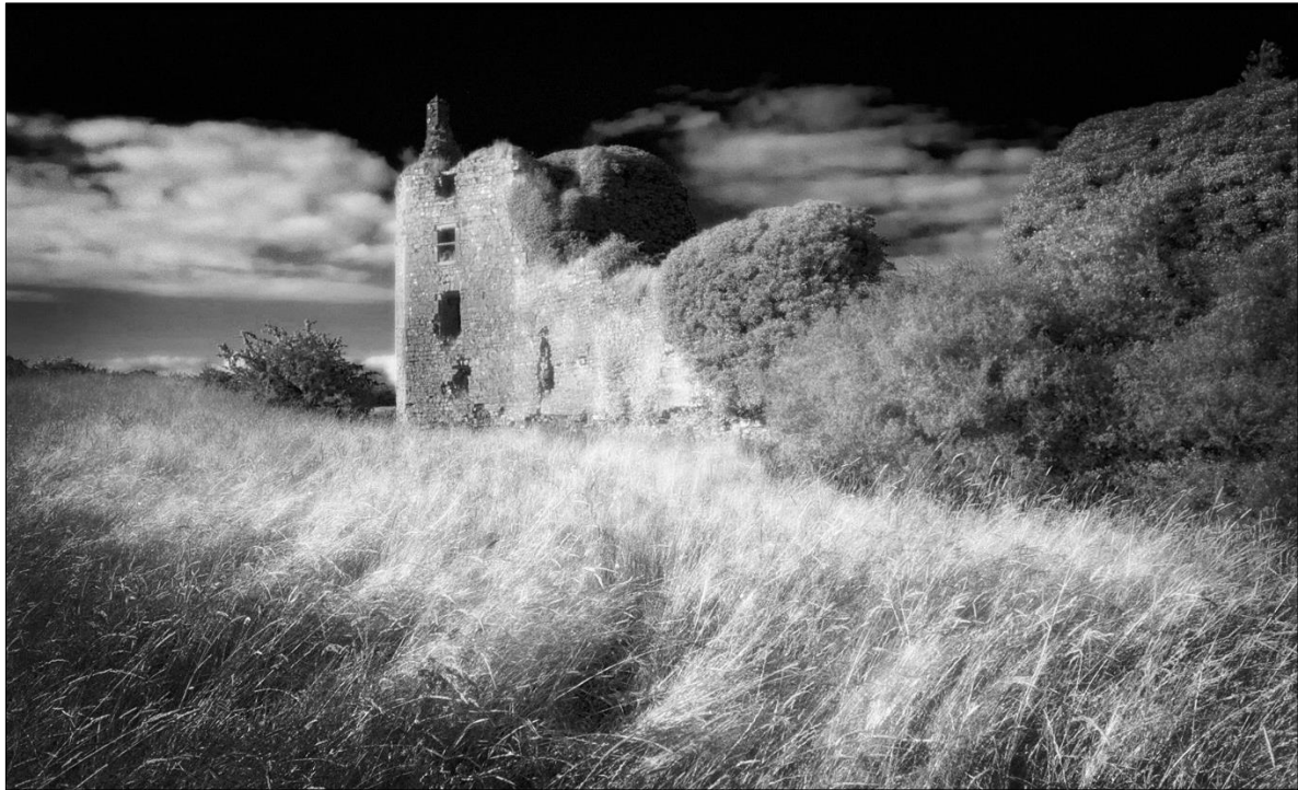
Plate 1: Ballintober Castle, from the Southwest.
