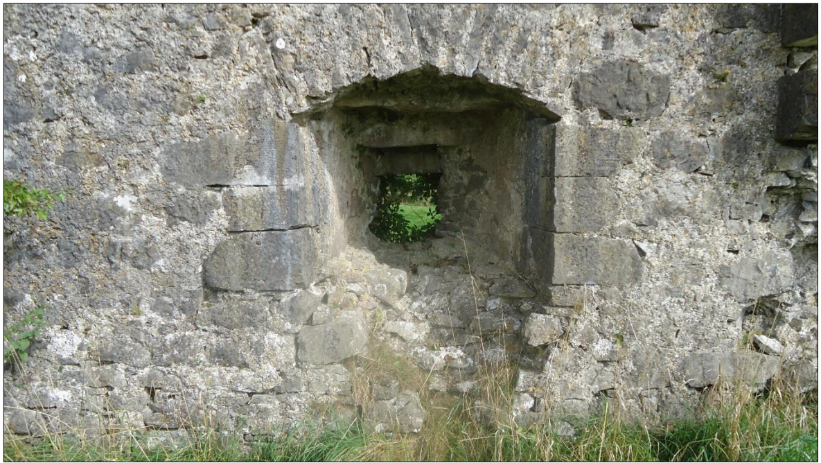
Plate 15: Ballintober Castle, view looking at interior of north wall showing gun loop next to mural stairs
