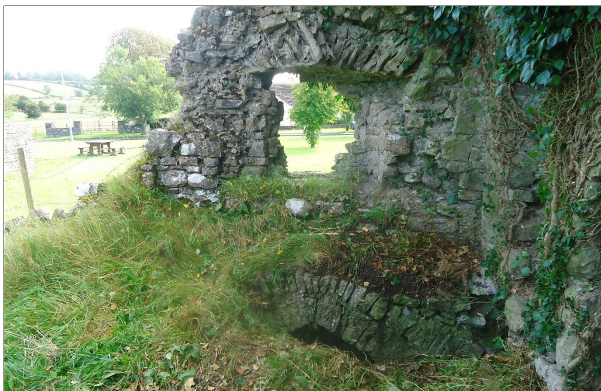
Plate 75: Ballintober Castle, eastern entrance, interior view looking East at ground-floor level, showing the basement arch extending below
