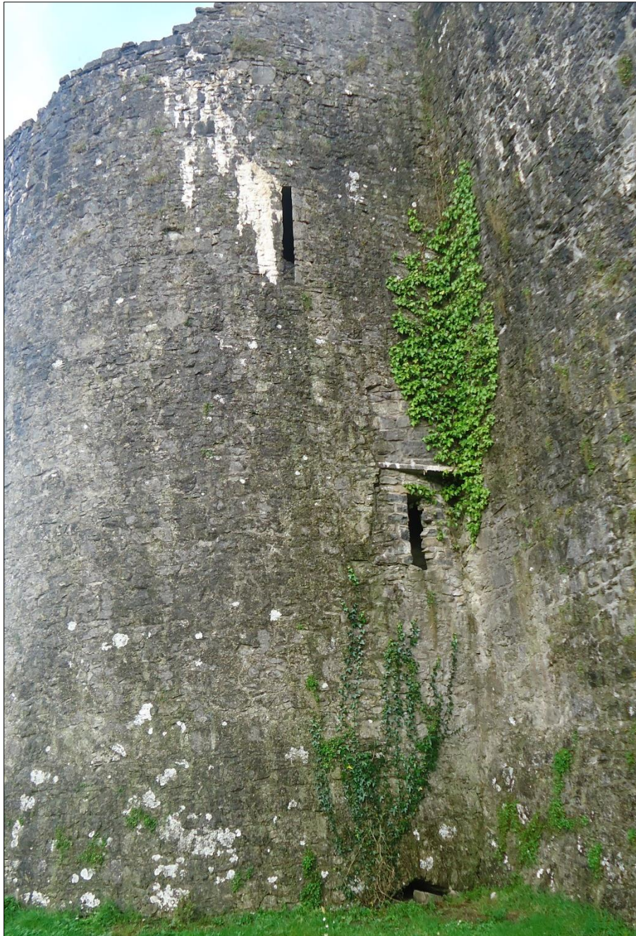
Plate 36: Defensive slit openings, Ballymote Castle. View looking Northeast at western mural tower, showing the tall arrow slits, to contrast with the much shorter versions at Ballintober.
