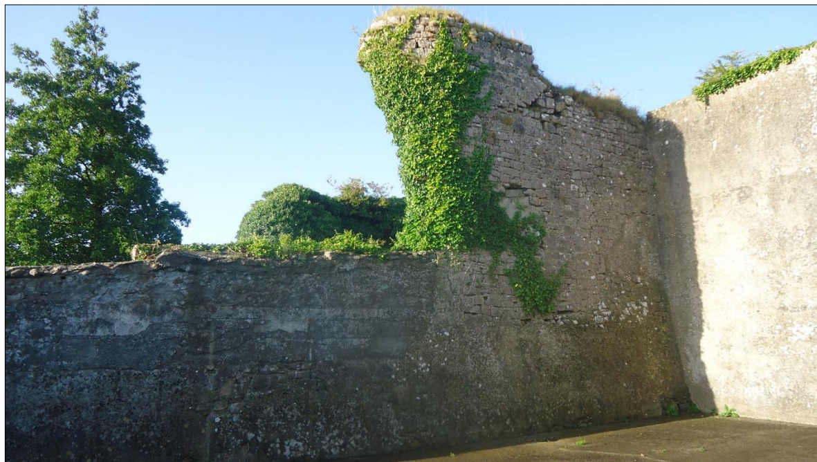
Plate 70: Ballintober Castle, eastern entrance, view from within handball alley showing the standing remains of the north tower. Note the steeply-pitched base batter that survives on the tower wall; it is one of few original elements of the castle's base batter that remains in situ
