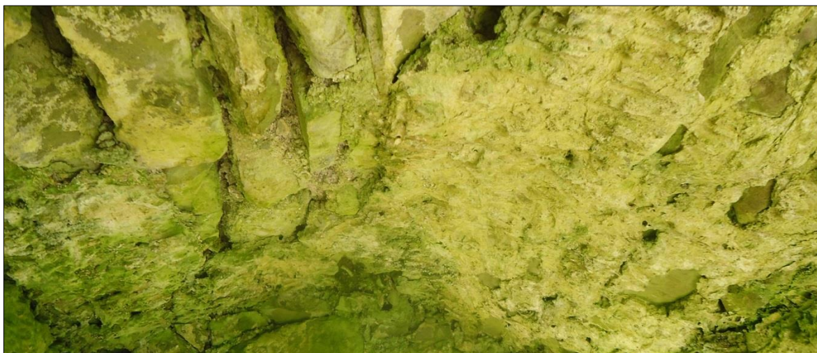
Plate 48: Ballintober Castle, northwest corner tower, detail of ceiling above entrance to first floor, showing remnants of wicker centring
