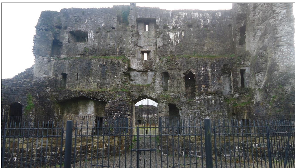
Plate 77: Entrance detail, Ballymote Castle. View is from the outside and shows the entrance at the centre, flanked by four-storeyed towers on each side, with the space between inhabited as part of the overall residential block. On a smaller scale, it is possible to imagine a similar arrangement existed at Ballintober Castle
