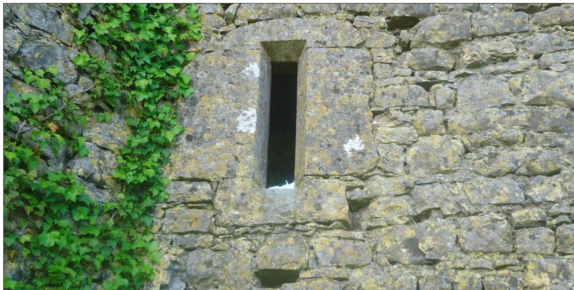
Plate 37: Ballintober Castle, northwest corner tower, view from outside looking at northeast-facing window on ground floor. These short vertical slits contrast with the defined arrow loops seen at Roscommon an Ballymote Castles in such locations (Plates 35-36)
