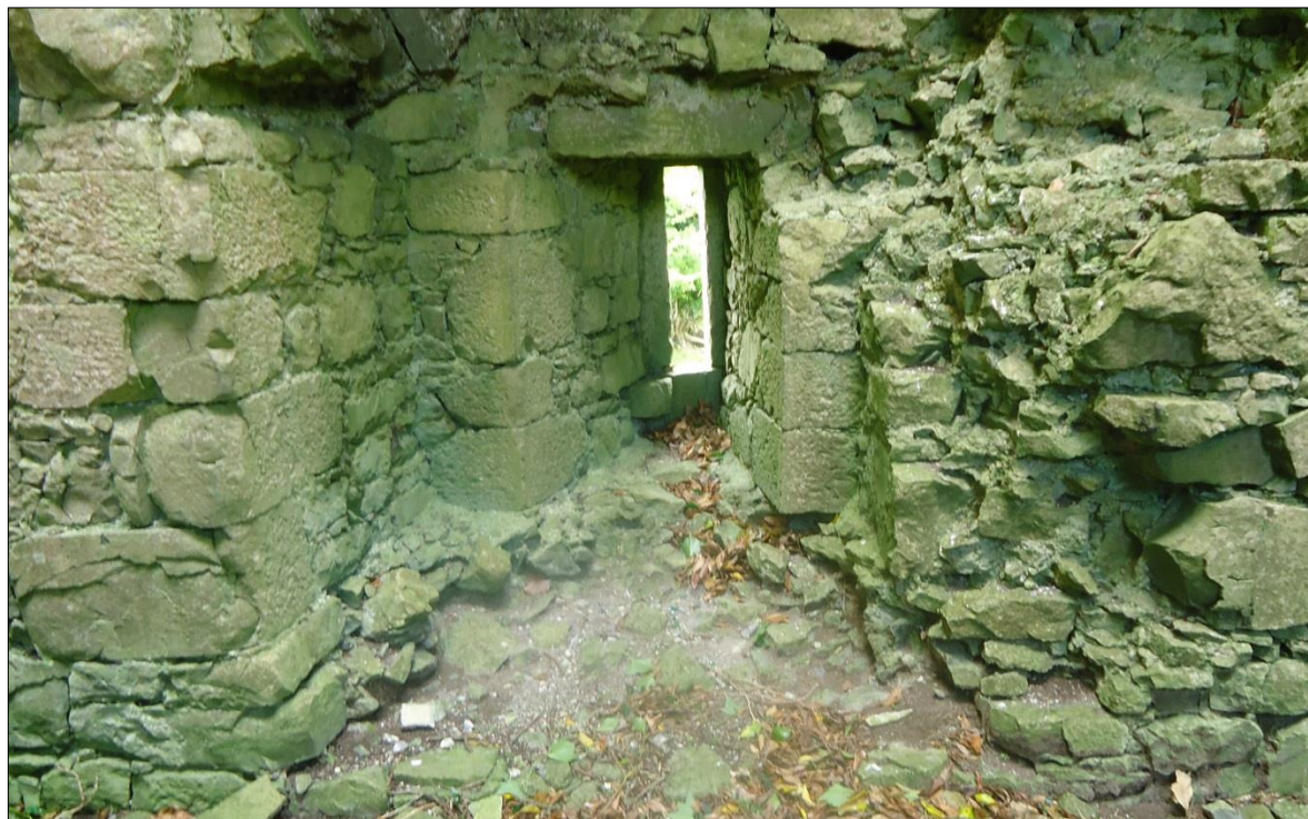
Plate 43: Ballintober Castle, northwest corner tower, view of the ground-floor window in the east wall
