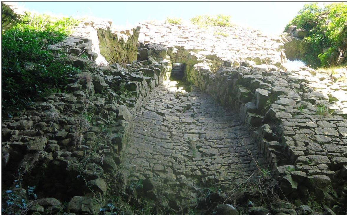
Plate 33: Ballintober Castle, southwest corner tower, view looking up to the fireplace on the first floor west wall. On the second floor above, the opening to the left (south) is a window and that on then right (north) is the entrance to the north chamber
