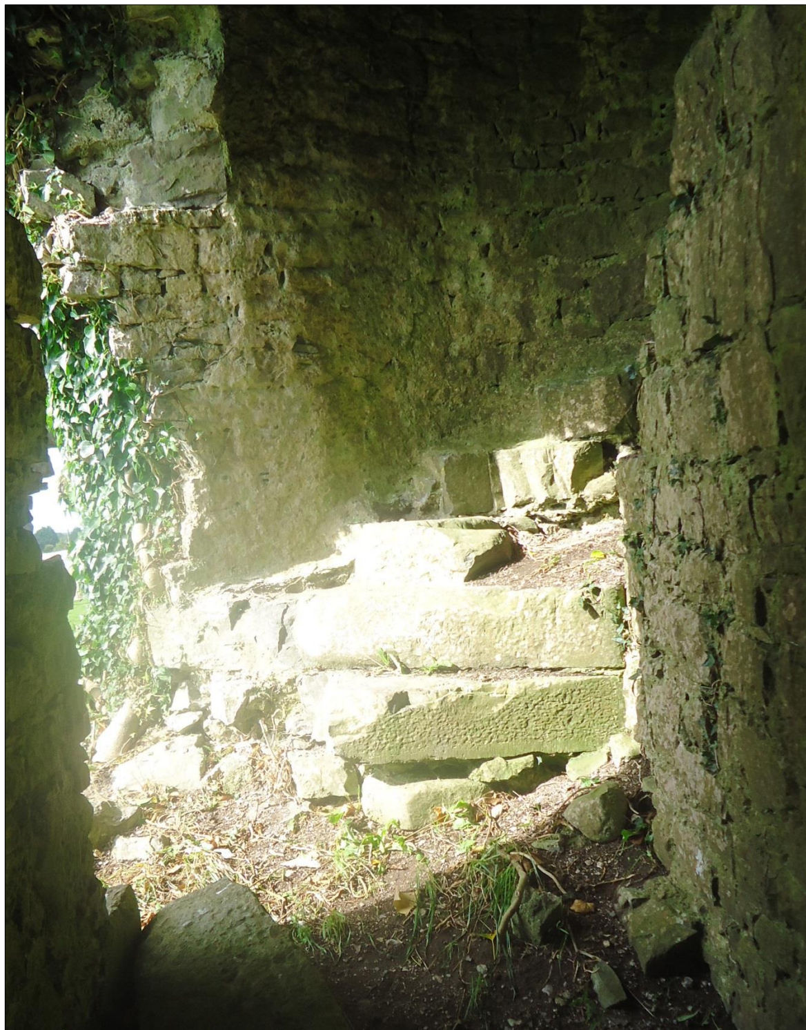
Plate 46: Ballintober Castle, northwest corner tower, view looking west to the base of the stairs
