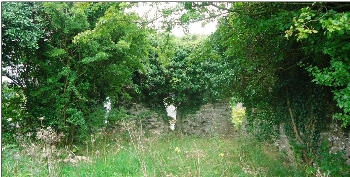
Plate 66: Ballintober Castle, southeast corner tower, interior view from the north
