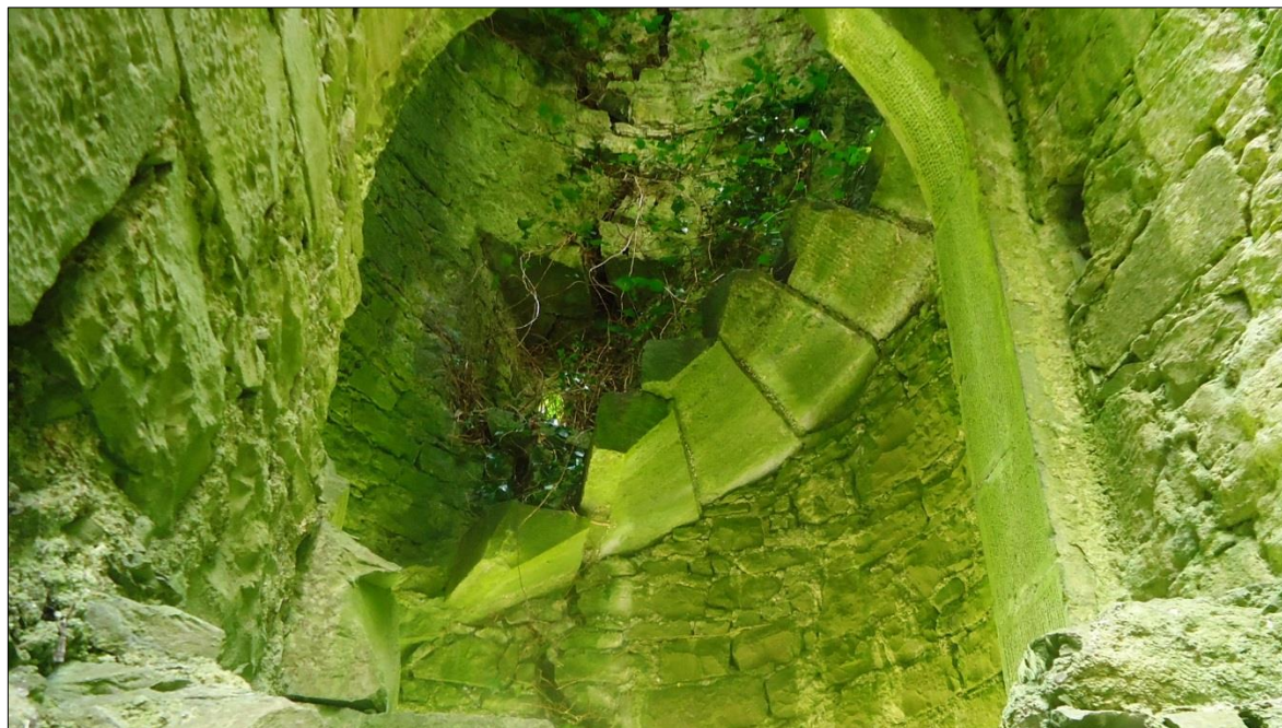
Plate 54: Ballintober Castle, northwest corner tower, view of the spiral stairs ascending above the first floor
