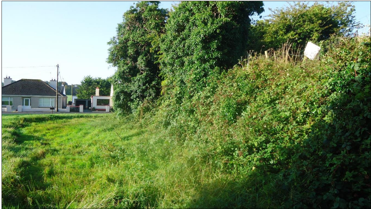
Plate 7: Ballintober Castle, view looking South of the fosse on the south side at the southeast corner
