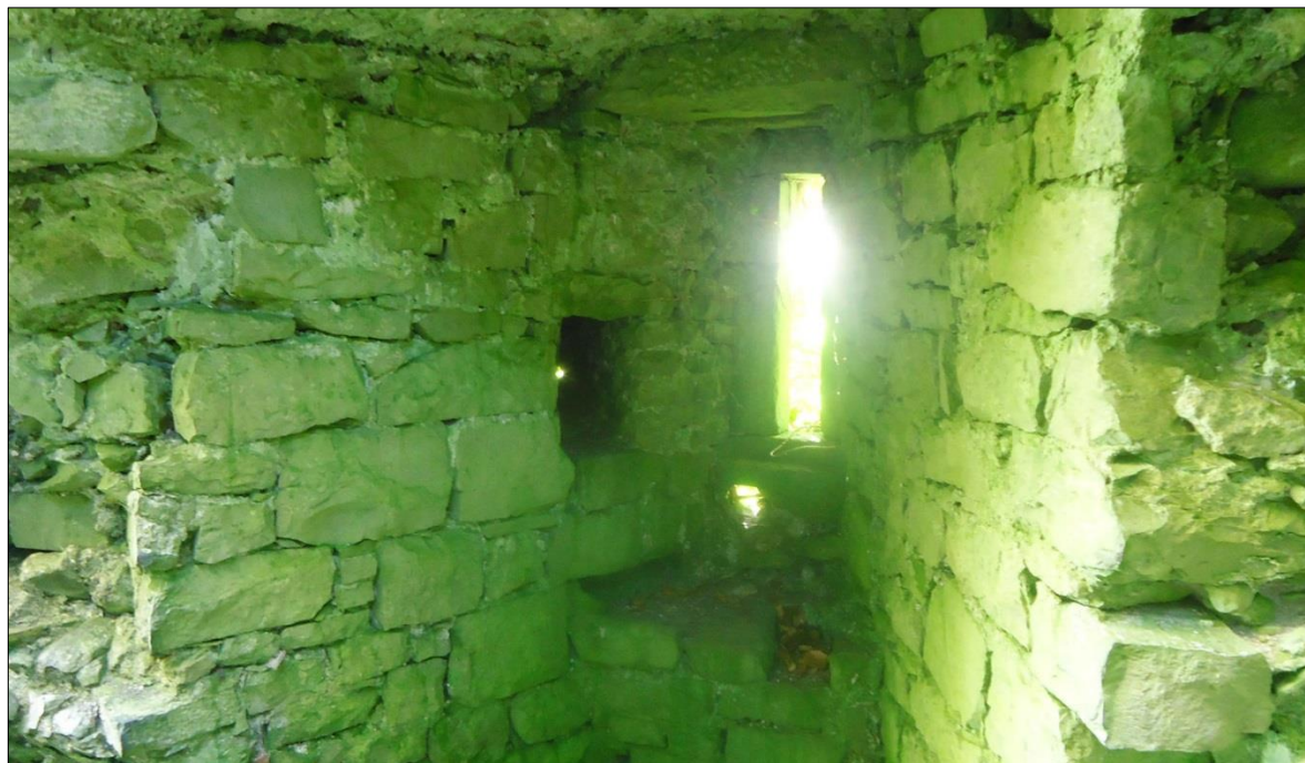
Plate 25: Ballintober Castle, southwest corner tower, view of the east window, showing second gun loop added on its north side
