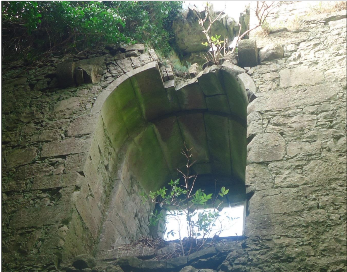
Plate 56: Ballintober Castle, northwest corner tower, view looking at the west-facing second- and third-floor windows from inside
