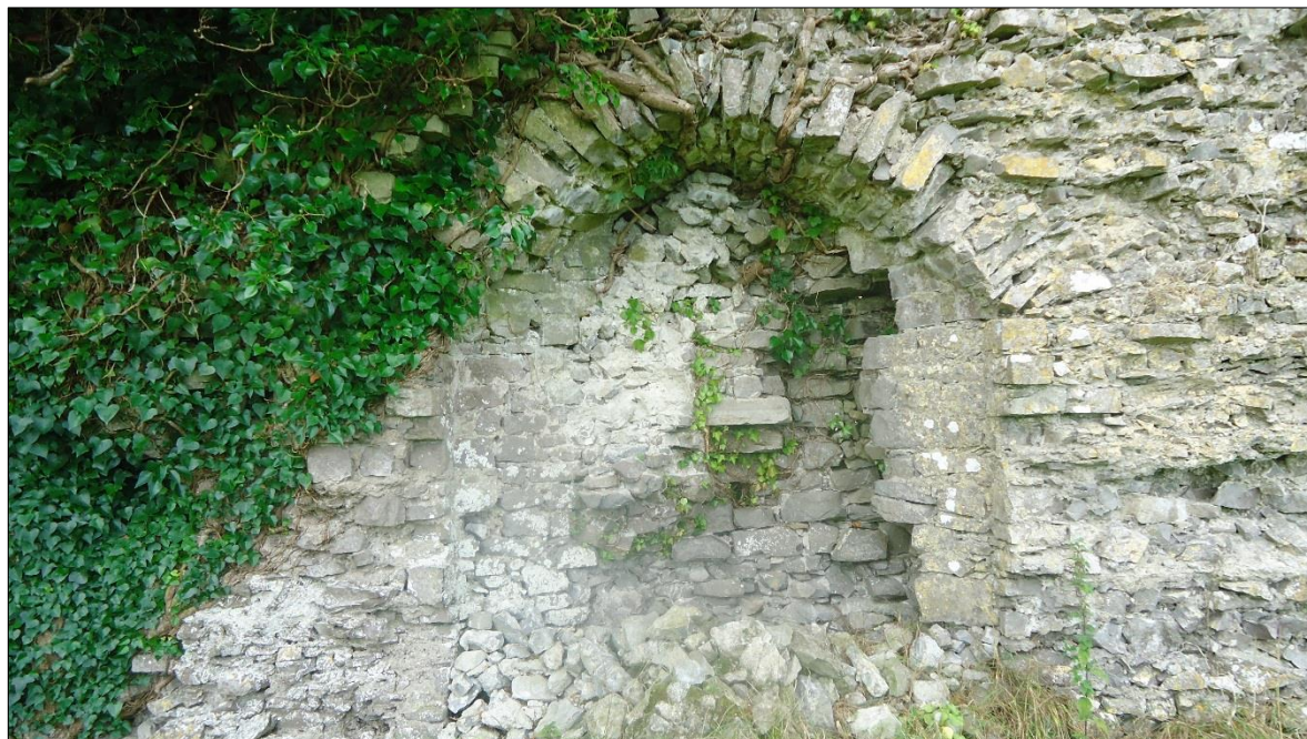
Plate 11: Ballintober Castle, view looking at interior of west wall on the south side showing window opening under arch
