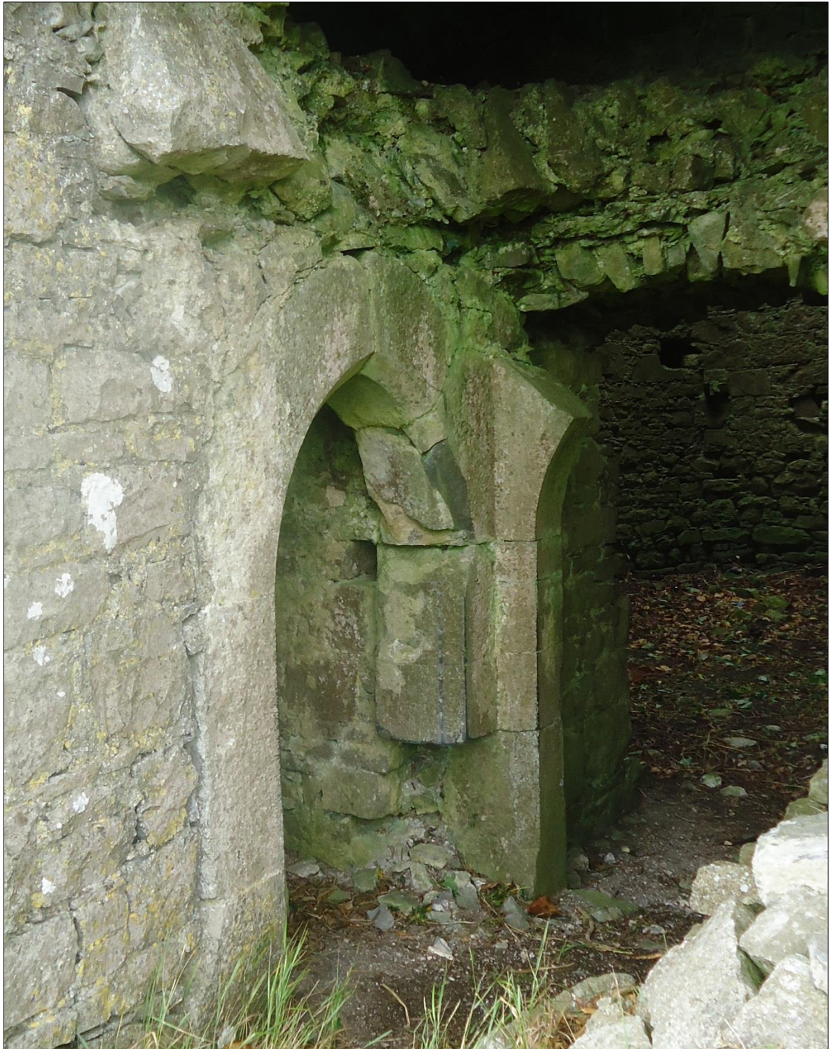
Plate 41: Ballintober Castle, northwest corner tower, view looking through entrance to two doorways, the left (West) leading to the stairs and the right (North) leading into the main chamber. The picture also shows the vaulting in the roof above, which has collapsed
