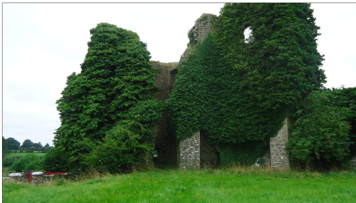
Plate 20: Ballintober Castle, view looking South at exterior of the southwest corner tower, showing the presence of two buttresses inserted to support the tower and the residential chamber to its north
