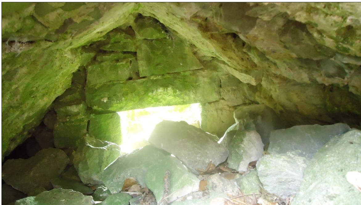
Plate 76: Ballintober Castle, eastern entrance, interior view of the basement level in the south tower looking East, showing the steeply-pitched roof, the window/gun-loop opening in the east wall, and the collapse that fills the chamber
