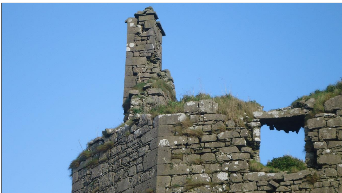
Plate 60: Ballintober Castle, northwest corner tower, exterior view of the roofline and chimney. Two dripstones are visible at the left (Northwest) angle at eaves level
