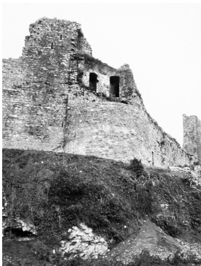
Figure 8: External view of the Westgate Tower during restoration, c.1930, from south (© Pembroke Castle Trust)
