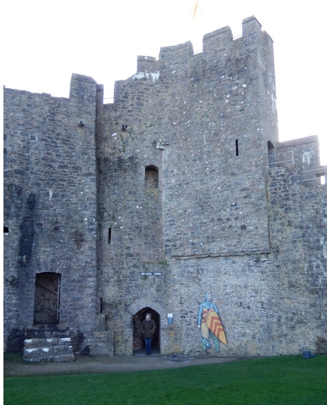
Figure 3: The rear face of the Westgate Tower, from north
