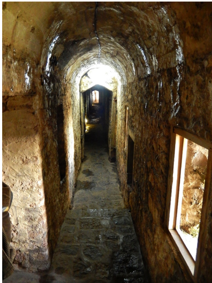
Figure 5: The mural passage just east of the Westgate Tower, looking east. The former latrine shaft lies beneath the square recess in the middle distance, on right, and is now represented by a small opening for a pipe
