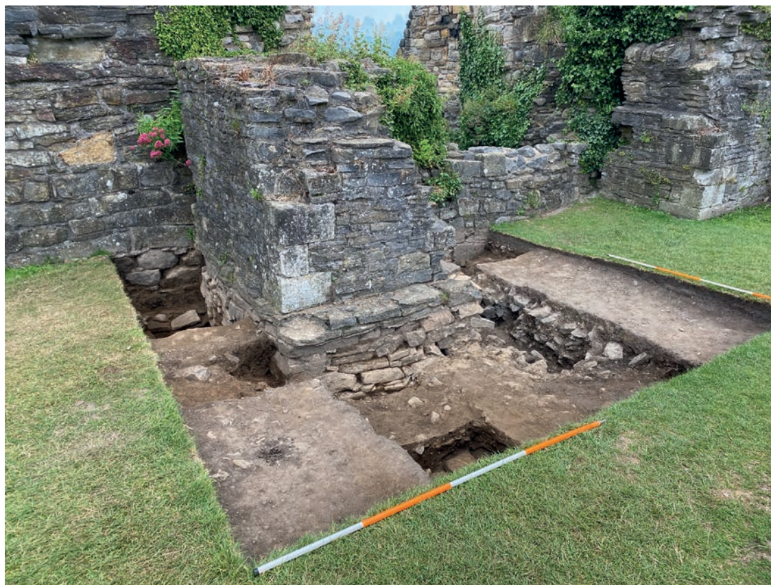
Figure 3. Overall view of Trench 1. The gap in the curtain wall is visible with the Ministry of Works wall infilling the gap. The difference between the medieval walling and the Ministry-created 'buttress' is also clear. Finally, the loosely compacted rubble fill of the former sally port ramp can be seen in section in the right-hand side of the trench
