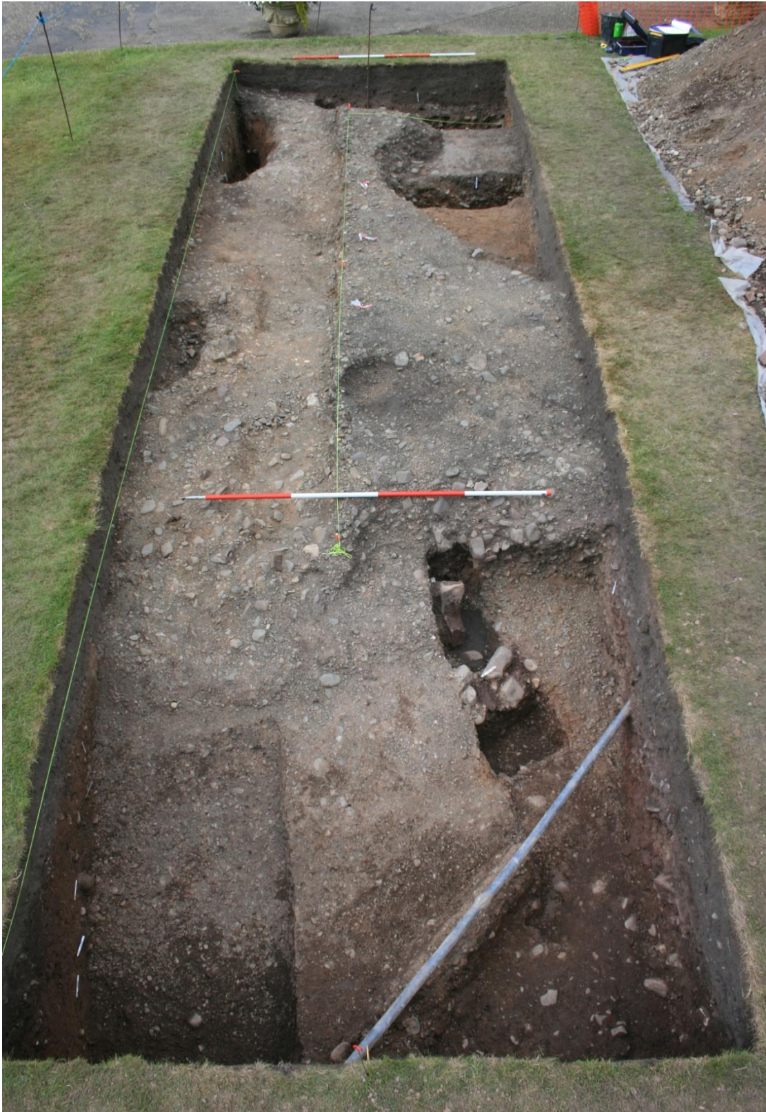
25 Final excavation view looking west, the slope of the motte ditch in the foreground, from the two-metre ranging pole. The ditch-fill deposits have been completely excavated only on the left side (south). Above the diagonal water-pipe are the probable post-hole 025 (excavated) and slot or gully 027 part-excavated in the foreground
