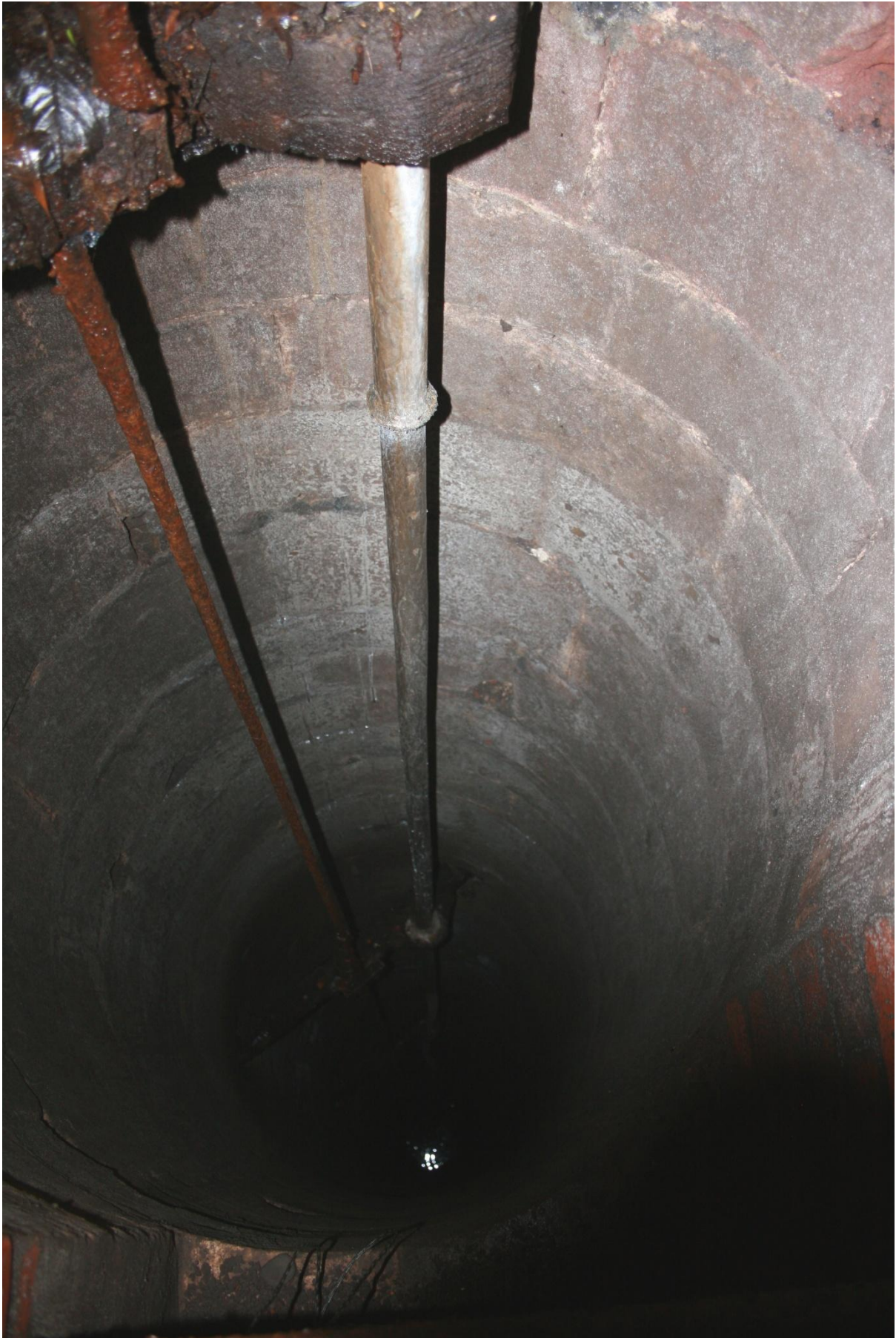
42 The well shaft. The light is reflecting off the surface of the water 21 metres down
