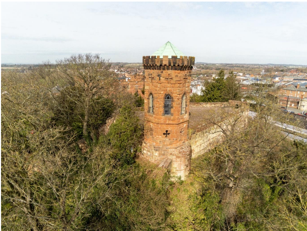
10. Drone shot of the motte from the south-east (James Brennan Associates). The watch tower base can be seen under Laura's Tower with the striped retaining wall beyond marking the making good of the collapsed side of the motte from the late 13 th century (James Brennan Associates)
