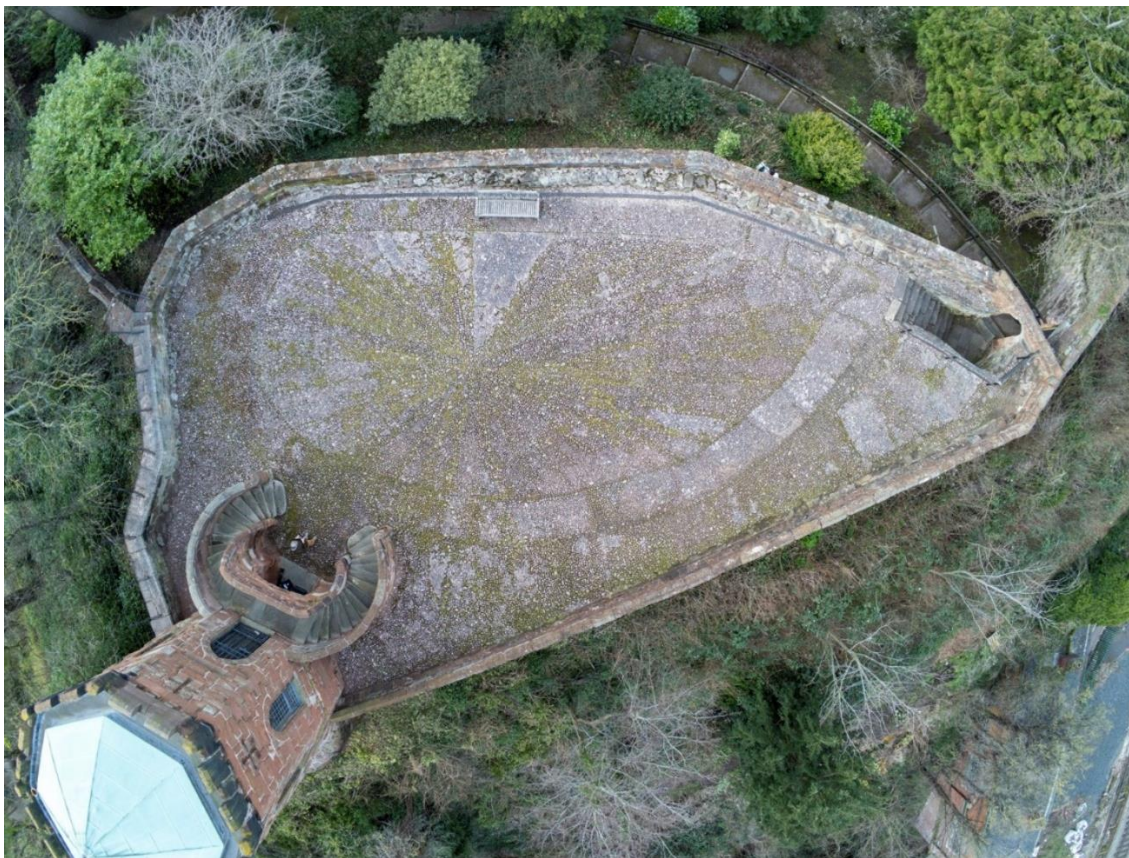
13. Drone photograph (James Brennan Associates) of the motte top in 2022 (north to right). The cobbled surface of the 1990s slopes down to the west (top) to shed water into the French drain running within the west perimeter wall and cutting through it at the SW angle. Telford's path to Laura's Tower is marked out in the cobbling
