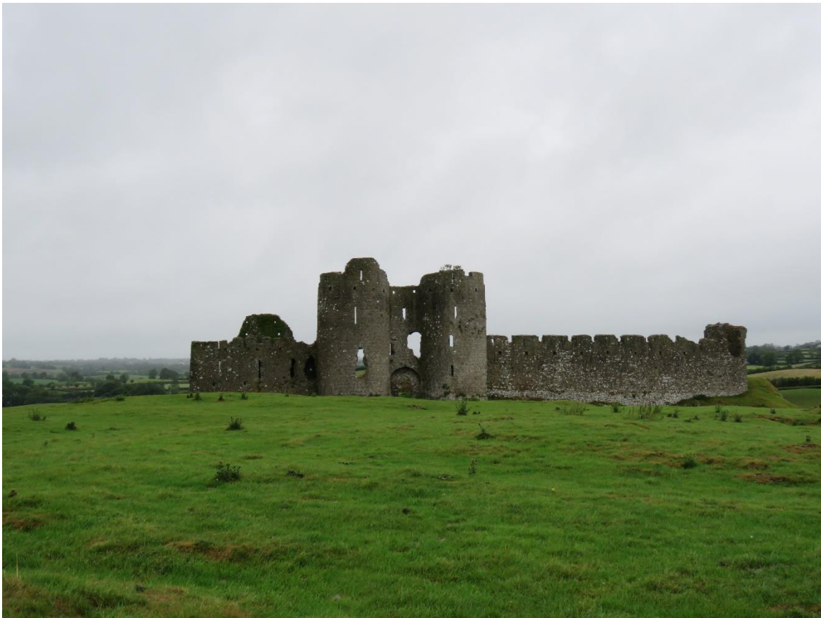
Figure 19 Castleroche, Co. Louth. View east across flat plateau
