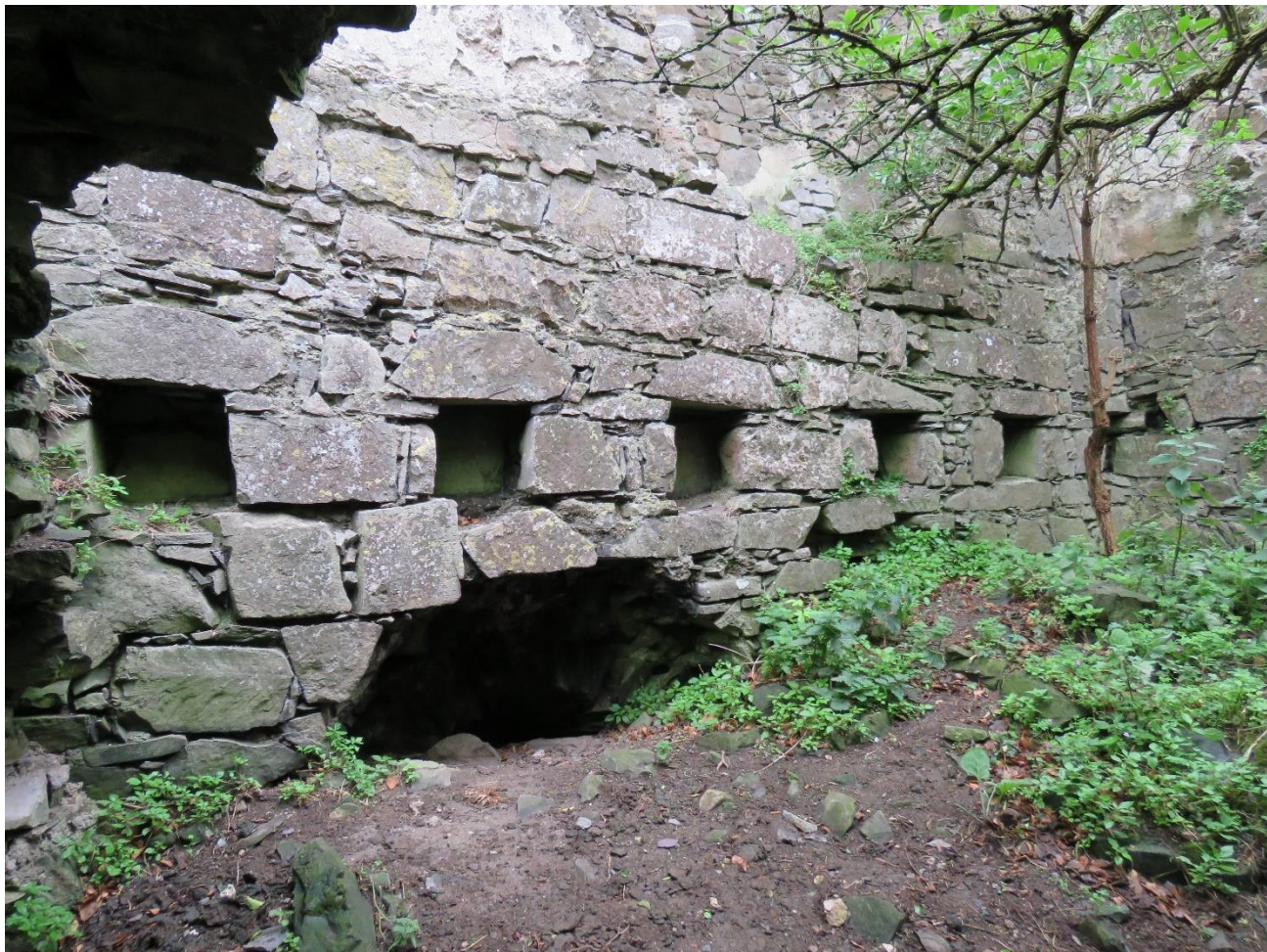
Figure 13 Interior of masonry chamber block facing east. Large putlogs holes plus thick masonry walls places this castle in the early thirteenth-century
