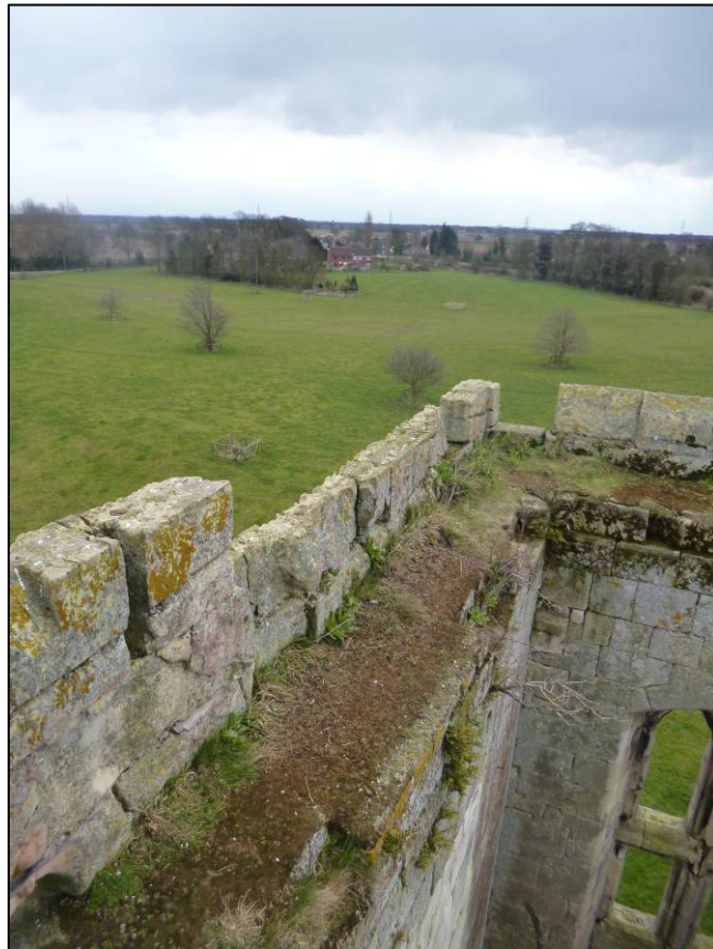
Plate 14: Parapet and wall-walk of south-west tower, looking S.
