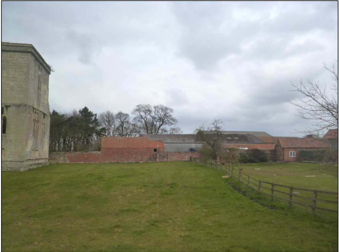
Plate 5: Area of gardens to east of south-east tower (Site 1c), with east moat to right (Site 2c), looking N.
