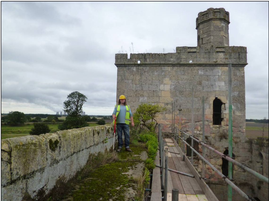
Plate 17: Parapet and wall-walk on south side of central range, looking W.
