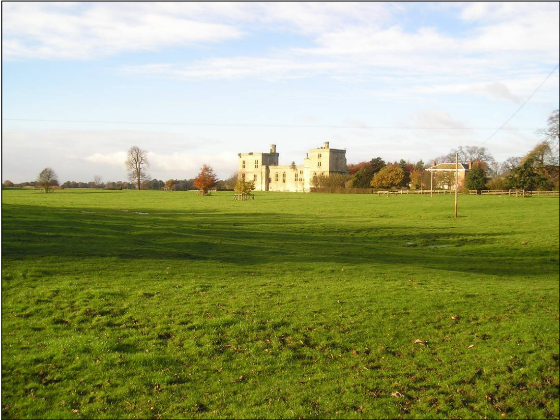
Plate 1: General view of EDAS survey area, looking SW.
