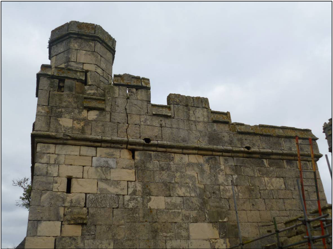
Plate 18: Crenulated parapet wall of south-east tower, showing original form, looking E.
